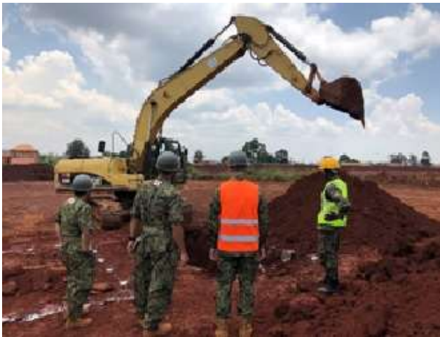
Excavating the soil by hydraulic excavator
