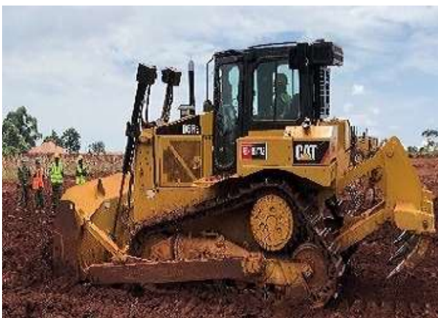
Using bulldozer to practice digging and moving the soil
