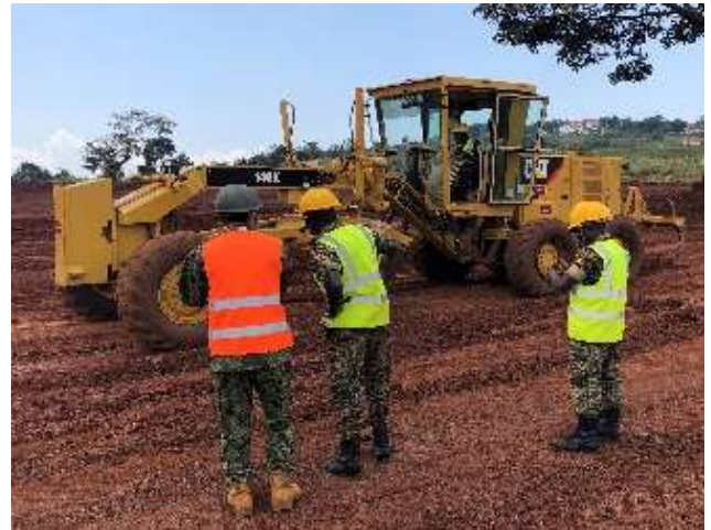
Practicing how to create ditch by grader
