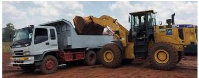
Practice of unloading soil from bucket loader to dump truck
