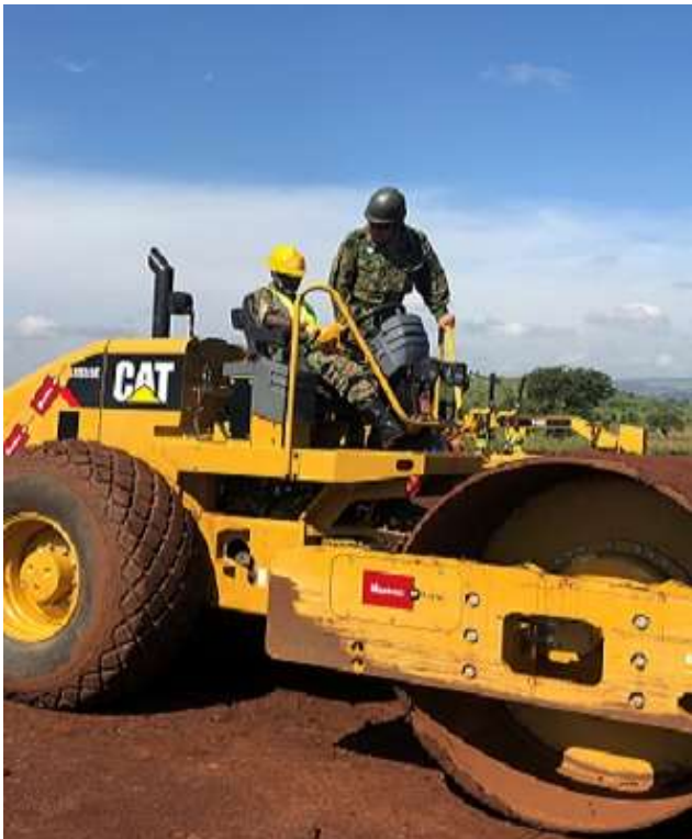
Teaching trainees how to compact the soil with road roller
