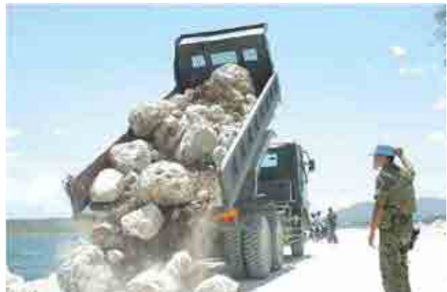
Japanese personnel at road repairing work
