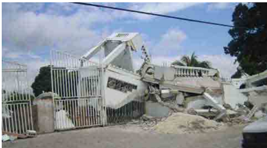
Collapsed building by the earthquake
