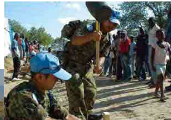
Japanese Personnel at ground leveling work at an IDP camp
