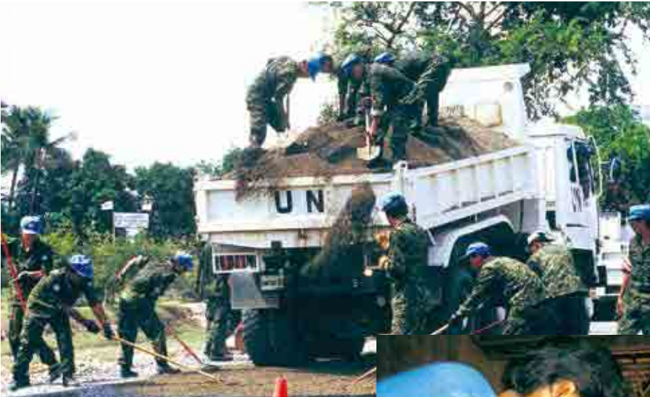
Repairing National Road 3
