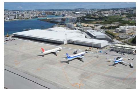
Naha Airport, International Logistics Hub
